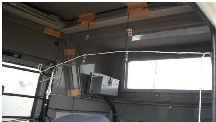
Figure 87: Equipment Installation in the Machine [3/4]
