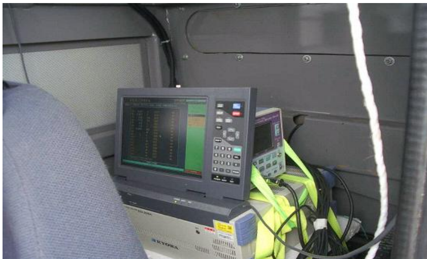
Figure 88: Equipment Installation in the Machine [4/4]
