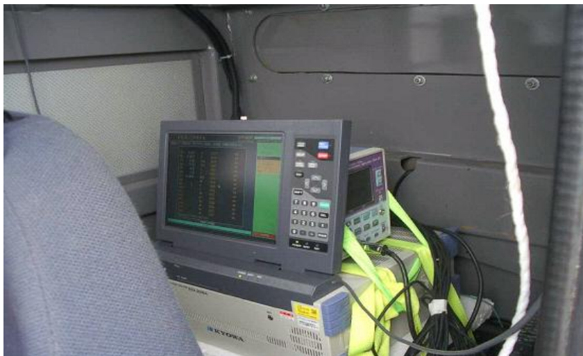
Figure 88: Equipment Installation in the Machine [4/4]
