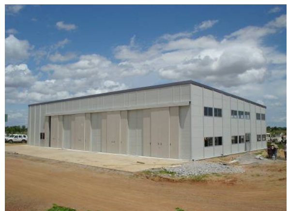
Central Workshop facilities in Battambang Province
